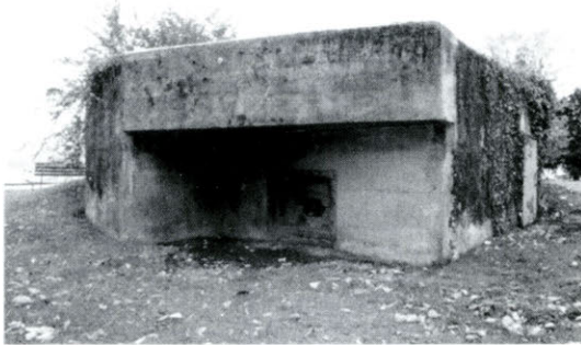
Bunker in Kilchberg
